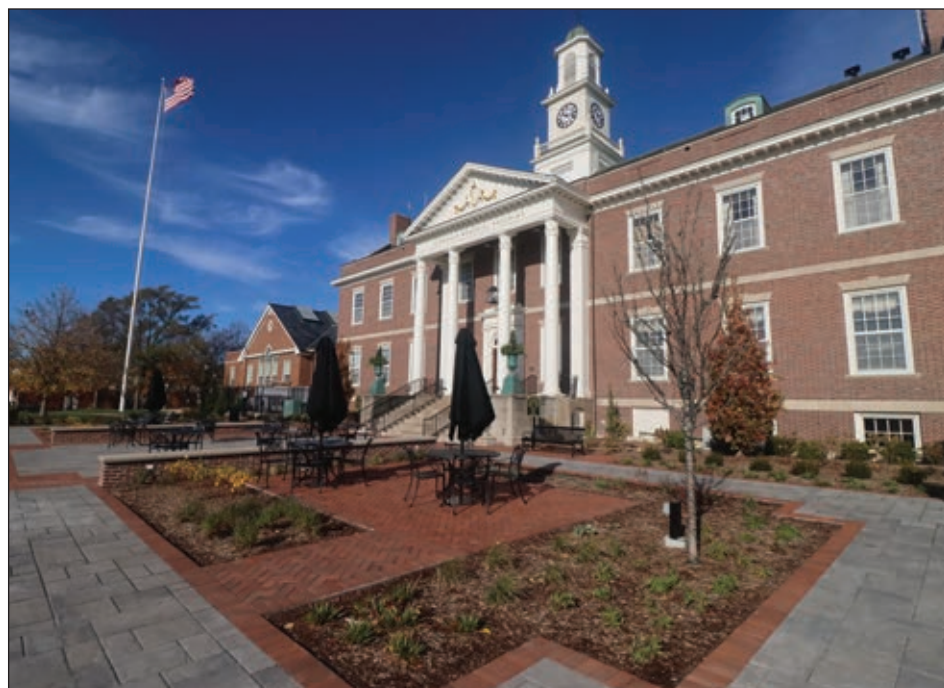
The renovated plaza in front of the Hinsdale Memorial Building will be the backdrop for many events, including library programs next year and the Hinsdale Christmas Walk Dec. 6. (Jim Slonoff photo)
