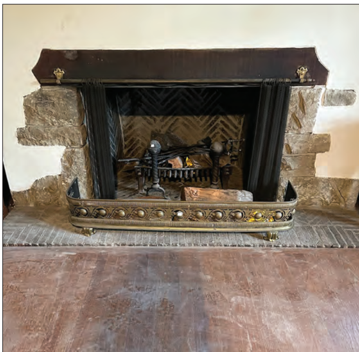
Hinsdale resident Mimi Collins has found numerous examples of Zook's design details while rehabbing 4 E. Fifth St., like the herringbone brickwork inside the living room fireplace. "He brought a charming style of architecture. People remember them," she said. (photo provided by Mimi Collins)
