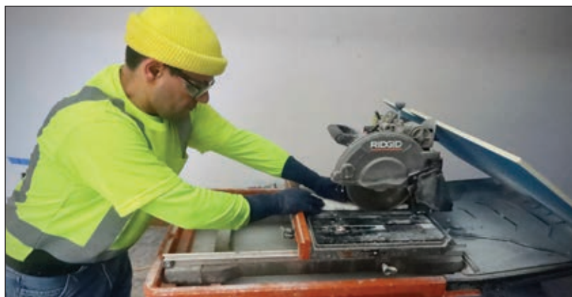
Subcontractor Tony Lopresti cuts tile and assists Piero Scoleri in laying it in the primary bathroom at 4 E. Fifth St. The previous space-deficient bath was enlarged, helping convert the historic home into a more livable one. (Jim Slonoff photos)
